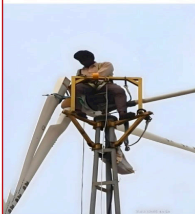
RIG FOR INSTALLATION AND UNINSTALLATION OF WINDMILL
